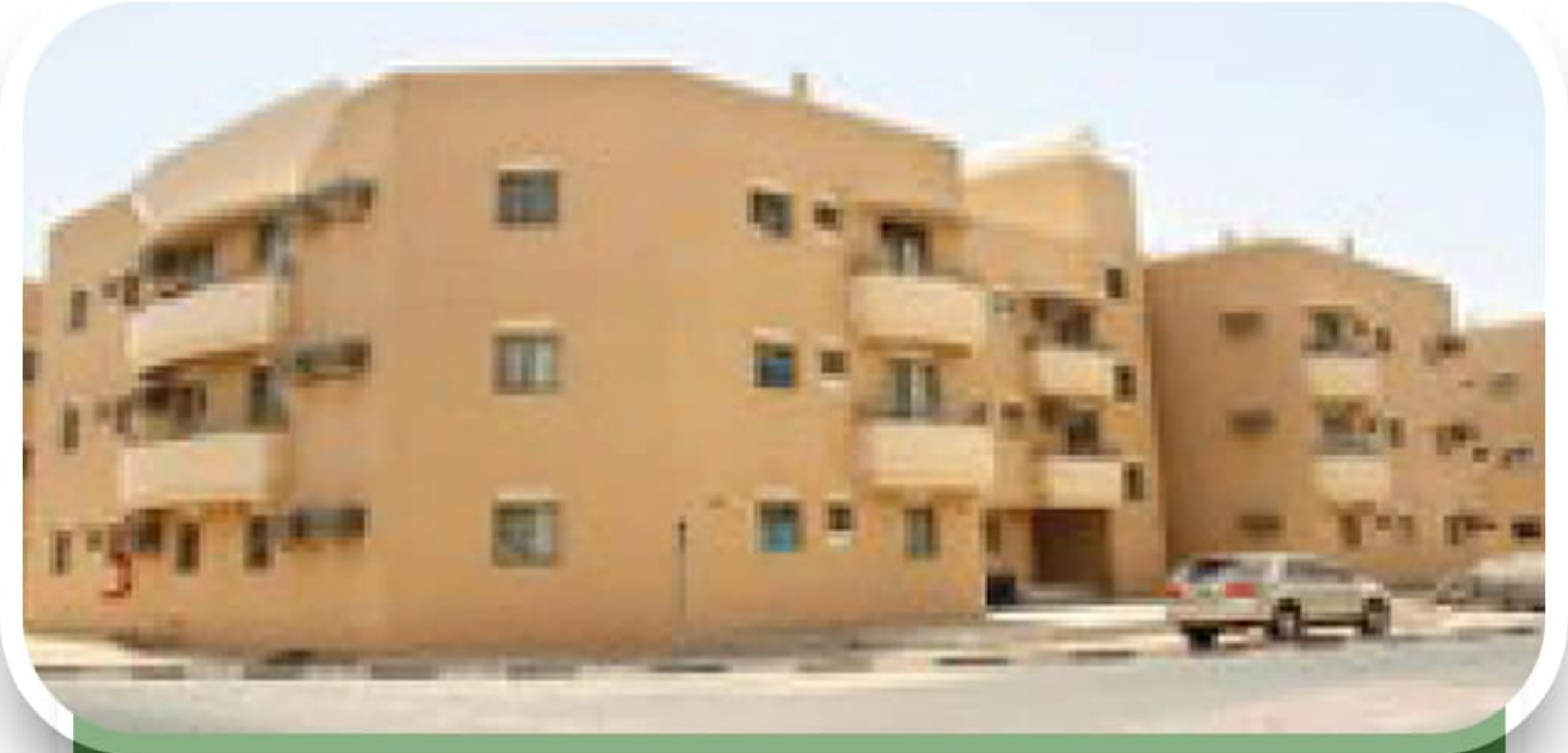
R327 F BLOCK BUILDING MUHAISNAH
