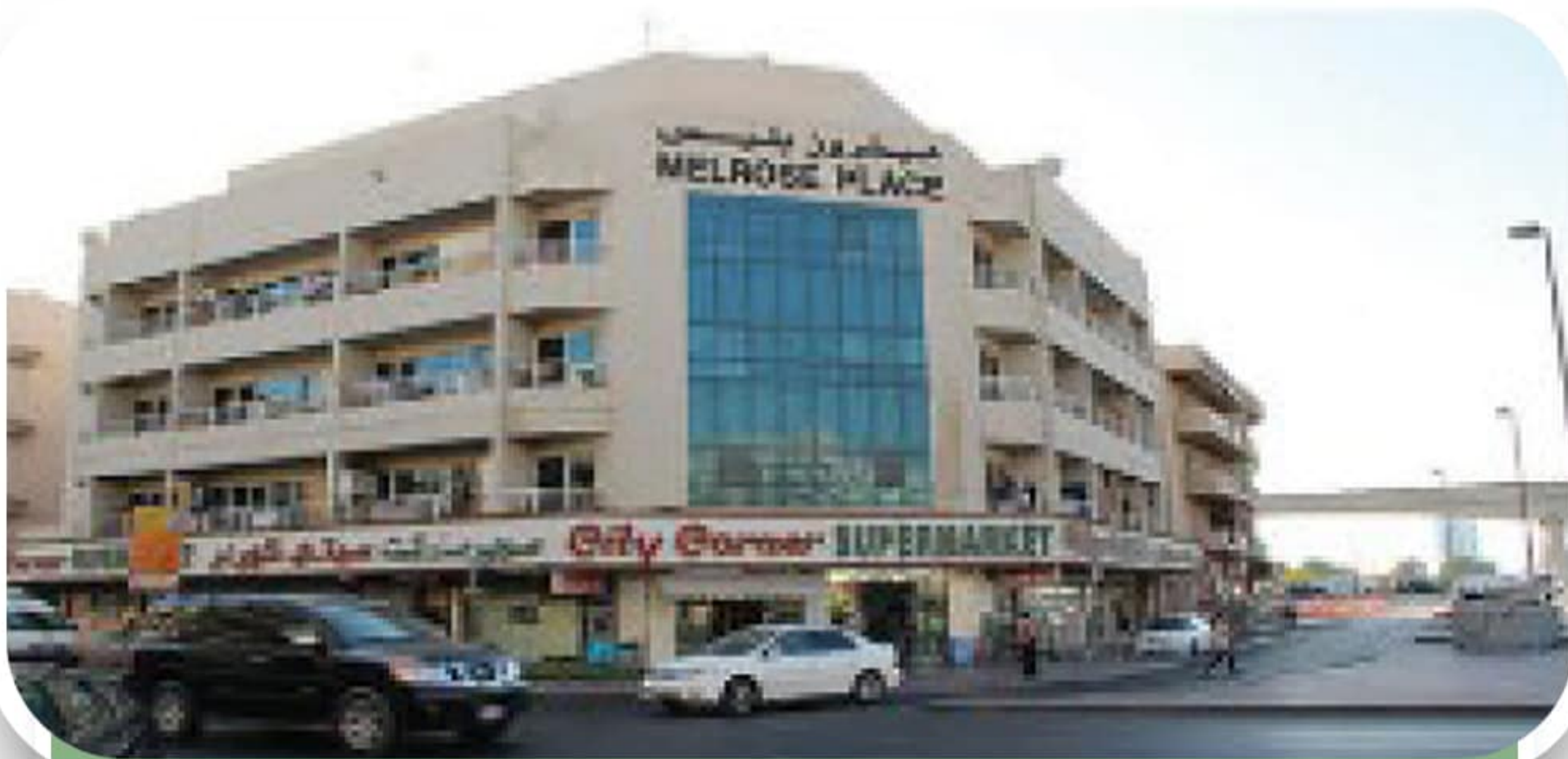
MELROSE PLACE BUILDING KARAMA
